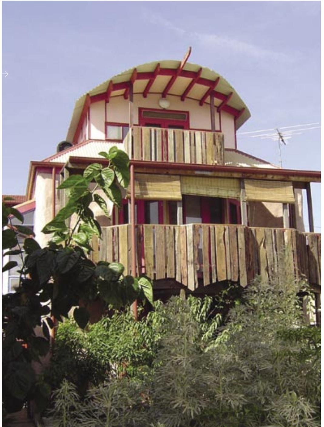
reused for paving and other decorative feature elements. Plantation pine was used for the joists, and many of the interior features were made from recycled timbers, such as the spiral staircases featuring steel, recycled jarrah and other Australian hardwoods.
